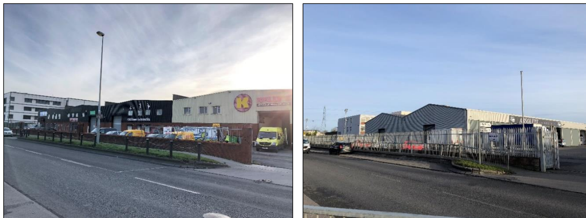
Figure 18.0 Existing view of the subject site as viewed from Cookstown Road (north) looking south (left) and Cookstown Road (west) looking east (right)
