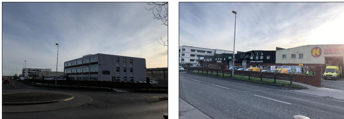
Figure 2.0 Existing view of the subject site as viewed from the intersection of Cookstown Road & First Avenue looking south-east (left) and Cookstown Road (north) looking south (right)
